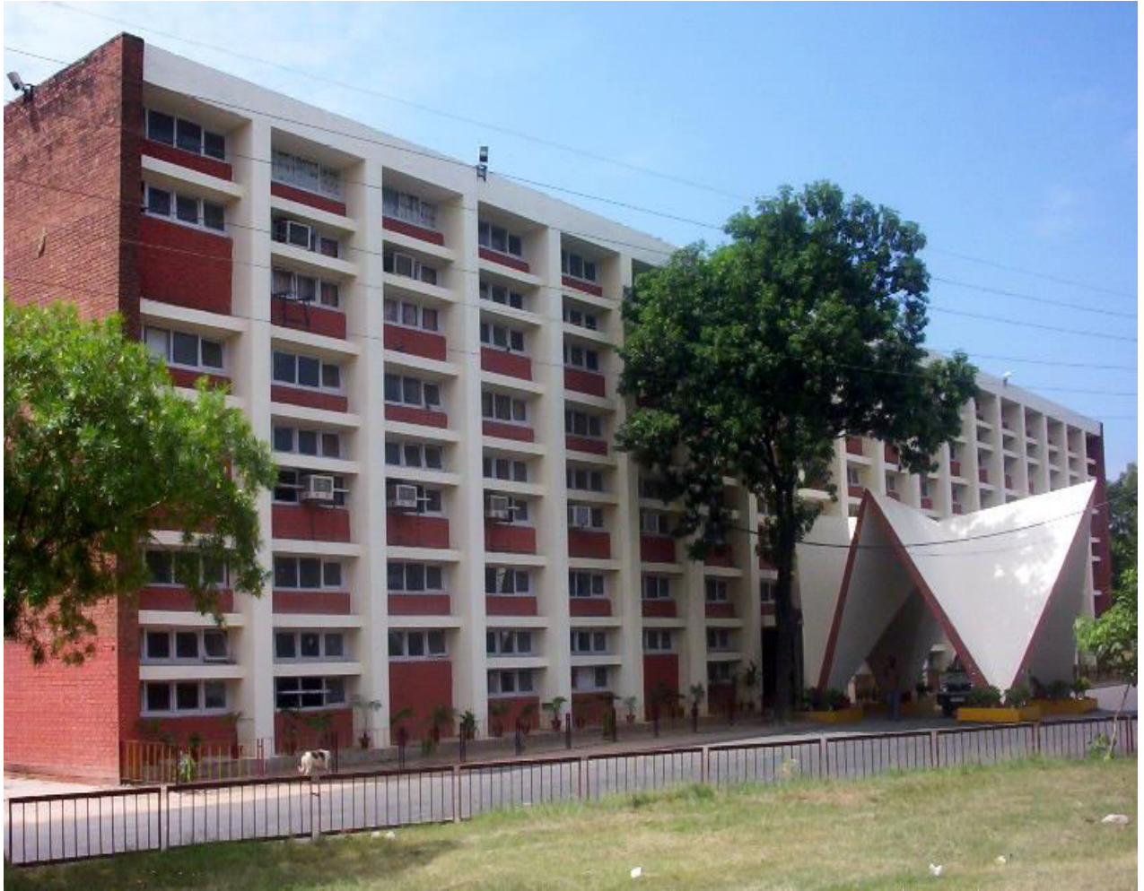
Building of Diploma Wing of CCET, Sector 26, U.T. Chandigarh
